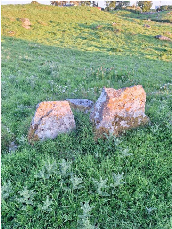
Figure B2. Upright and partly embedded stones with low relief continuing through the pasture. The arrangement may represent a relict boundary or structural feature, but requires expert inspection.
